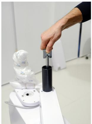
Tape the cables dentist panel and run them through the the post to cuspidor block with help of attached-bowden.
